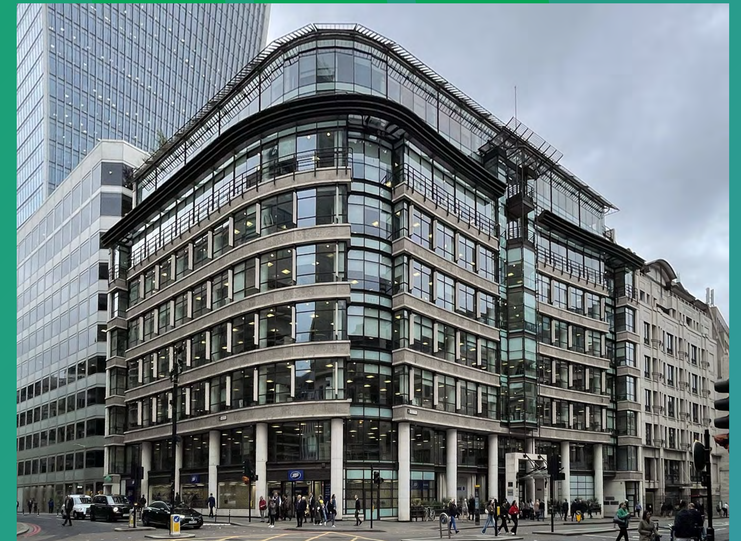
The existing building
