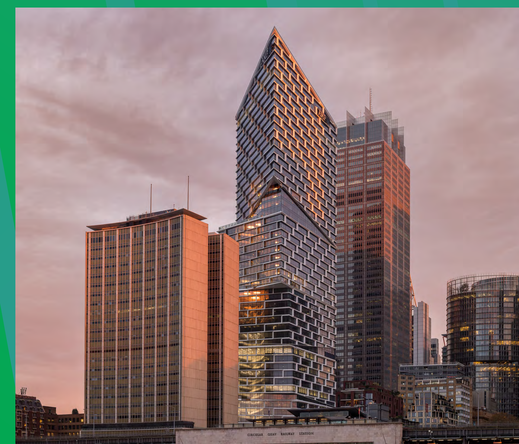
Sydney's Quay Quarter Tower
